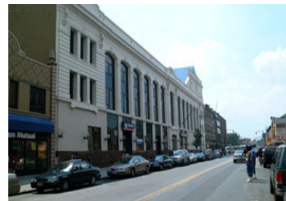
Preon receives a LOI for 3 TA100 microturbines in CHP applicaiton for Restoration Plaza—project will be on line late 2010.
