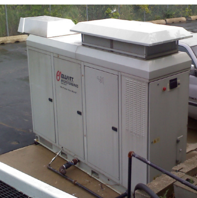
TA100 rich-burn microturbine provided by Preon undergoes independent third party validation of catalyst gas blend by Greenhart Engineering
